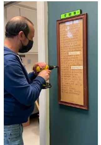
Ephraim secures the fire box code sign in the hallway
