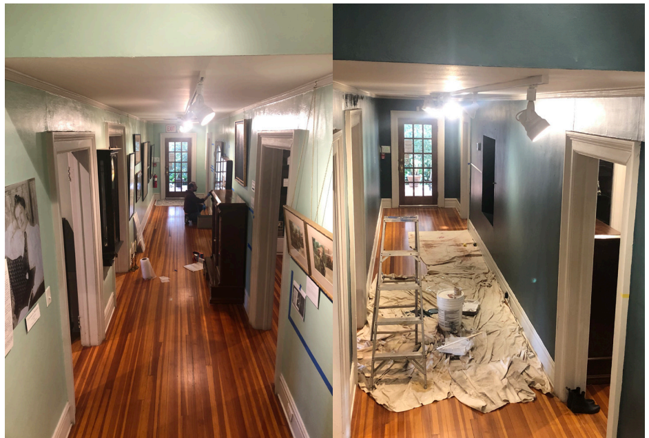
The main hallway before and during the transformation.
