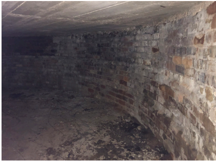
Ruins of the Ewart House foundation.
