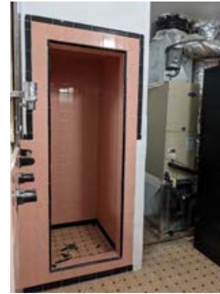
The shower stall before demolition.
