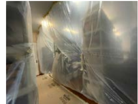
Plastic sheeting protected the collections during the renovation.
