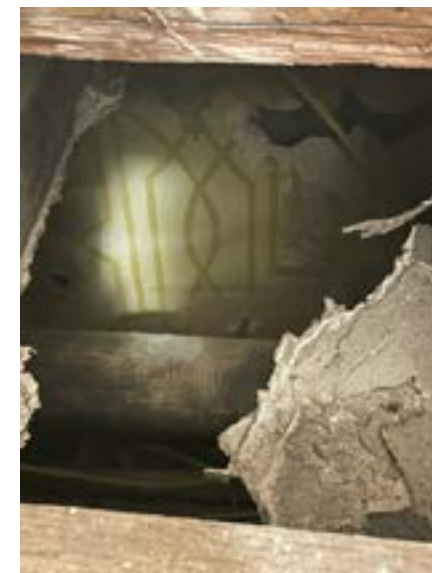
A glimpse at the re-discovered wallpaper through the floor joists.
